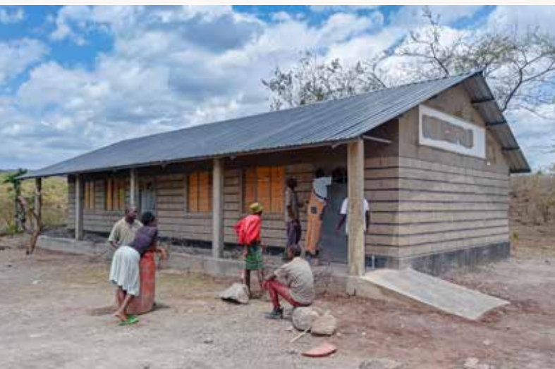
The classrooms of the new primary school in Lapoin
